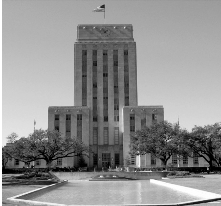
FIGURE 15: New Deal Civic Building City Hall, Houston, Texas
